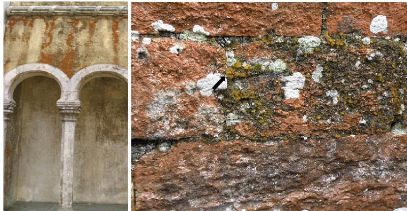
Fig. 9: The extended colonization of anthropogenic substrates by Trentepohlia species on the wall of the Palácio Nacional de Pena in the Portuguese city of Sintra (Macedo et al., 2009); building blocks at Mayan monuments of Becán in the Mexican state of Campeche (Ortega-Morales et al., 2013)
