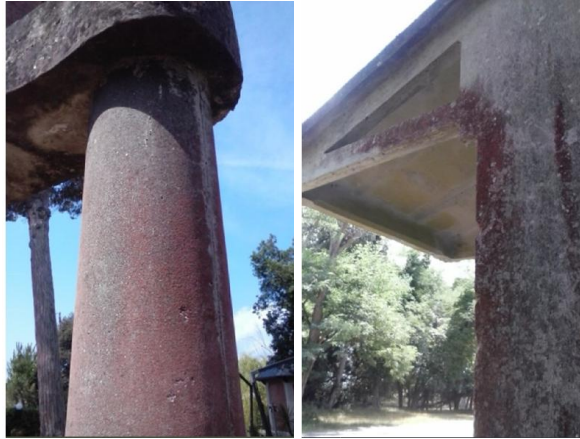
Fig. 11: Red stripes of the T. umbrina biofilm on some concrete constructions in Tirrenia (left) and S. Rossore Natural Park (right) in Pisa, Italy (photo by M. Šafránková, July 2015)
